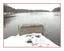
The smaller monument, Tri-State Rock, marks both the northwest end of the New Jersey and New York boundary and the north end of the New Jersey and Pennsylvania boundary. It is a small granite block with inscribed lines marking the boundaries of the three states and a bronze National Geodetic
