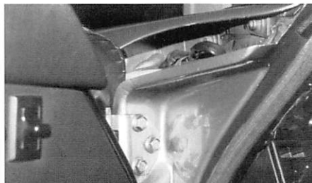
Remote location make the socket head screws challenging to loosen.
